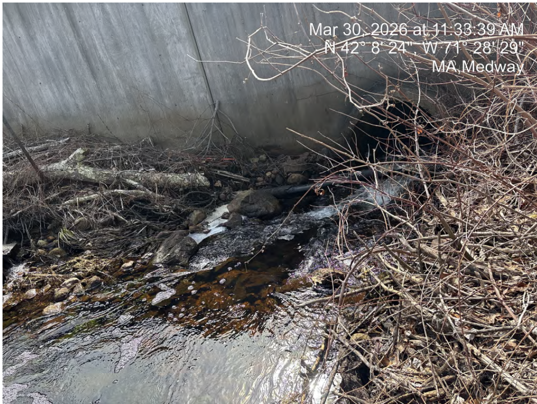
Photo 2. Photo of Stall Brook and the culvert adjacent to Alder Street facing south.
